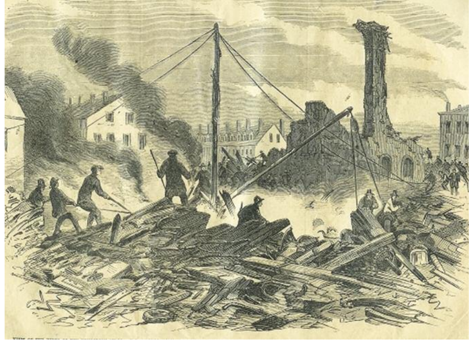
This newspaper illustration from the time shows the collapse of the Pemberton Mill in Lawrence.
