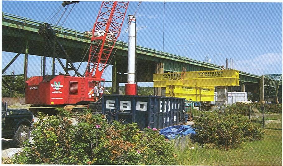
were still concerns about whether or not the tie-downs could hold such a large capacity and how they would react in that soil condition. Two tie-downs were installed and tested to the desired load. Production installation was monitored such that the tie-downs were installed using uniform or consistent grout volumes and water pressures.
