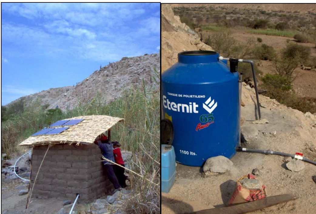
Figure 1 Solar powered water supply system in Muchipampa, installed Jan. 2006
