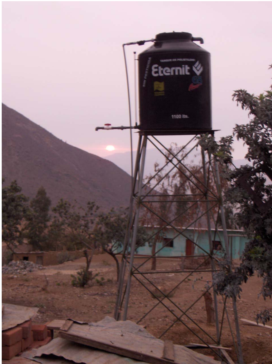
Figure 2 Tower and tank in Raypa, Jan. 2006
