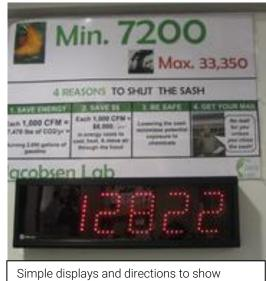
Simple displays and directions to show exhaust air flow rates and users' impact in fume hood driven spaces. The graphic above is from Harvard University's Jacobsen Lab.
