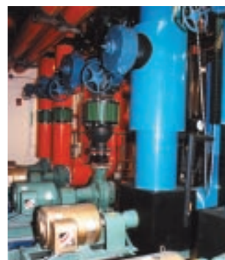
Heating and air conditioning machinery is housed in three separate areas of the building and is computer-controlled.
