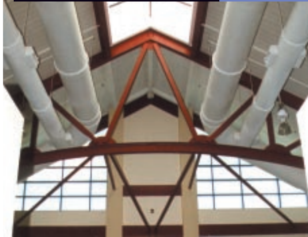
The building was designed with long span steel trusses and huge windows that create an atmosphere of light and airiness.
