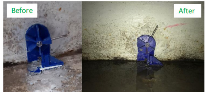
Performance of the displacement-monitoring indicator operating at the base of a wind turbine tower's harsh environment.
