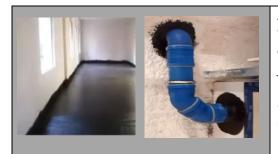
Air seal the interior with a permeable air barrier. Gypsum plaster works quite well combined with tapes and airtight paint, but other fluid applied vapor permeable air barriers will also do the job nicely. Air sealing must be done on both walls and the intersections of the intermediate floors to the exterior wall, across the ceiling and slab, at all rough openings and on all service penetrations.
