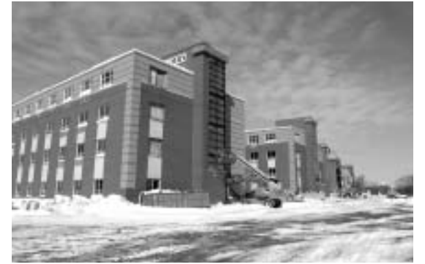
▲ Construction is nearly complete on the six new Lawrence High Schools.
