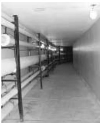
▲ The University's tunnel system, constructed originally to carry steam and other utilities from building to building, is a popular pedestrian way for students, staff and faculty.
